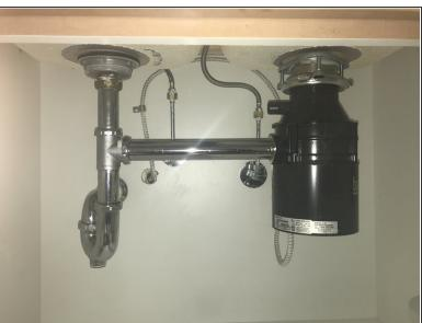
Shut off valves that are located under the sink and position faucet in the center to drain remaining water.
