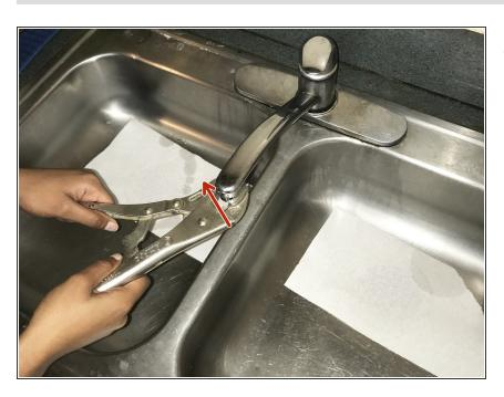
Unscrew and remove aerator with a wrench.
