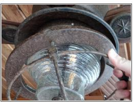
Make sure no power is flowing to the fan. Then begin by removing the metal light frame by twisting.
