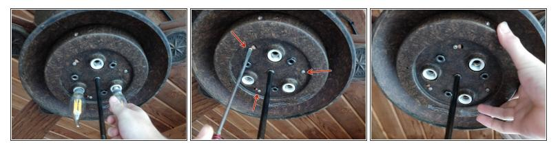
Remove lightbulbs to avoid damage when removing light pan. Then, remove all three fitter plate screws. This will cause the light pan to hang from the electrical wires.
