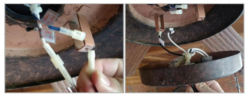
Disconnect single pin connectors to finish removing light fixture from fan.
