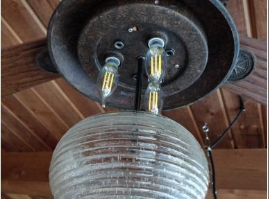
Unscrew the finial (cover at the bottom of the glass globe). Then unscrew the hex nut and remove
