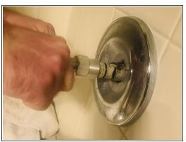
Once the valve comes out, you may experience some water coming from the shower socket opening; inspect the socket opening for any debris (rubber, slime, etc) that might be left behind after removing the cartridge.
