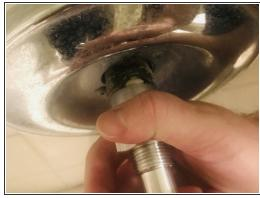
Use the Posi-Temp Puller to remove the cartridge from the shower; you'll need to screw it in place, then manually pull the cartridge out of the shower socket using a slow/controlled slightly twisting movement.
