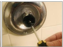
Take a Phillips head screwdriver to remove the handle adaptor and set it off to the side exactly how it was configured when it was attached.
