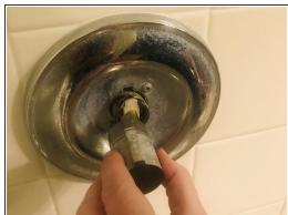
Pull off the collar to expose the valve cartridge that needs to be replaced.
