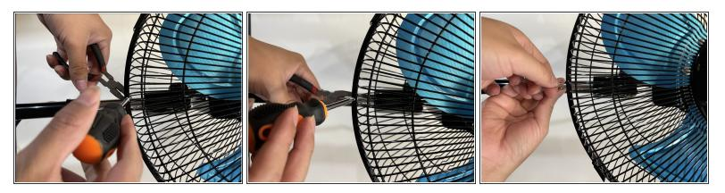
• Remove the single 0.8 mm screw using a Phillips #2 screwdriver. Use a pair of pliers to hold the hexagon nut so that it makes the process easier.
