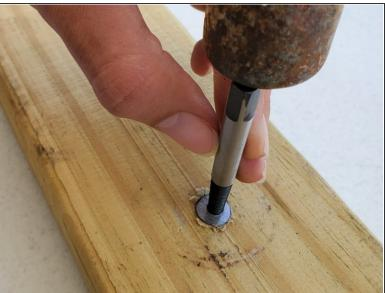
Insert a screw extractor in the hole and then hammer it inside, making sure it is tight.
