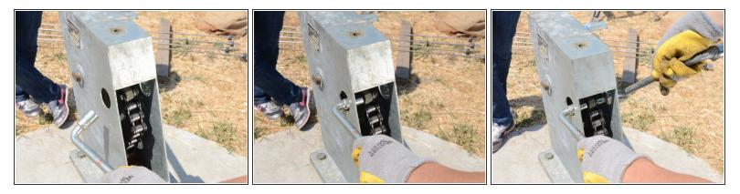
Using the two access holes, place an angled socket wrench on the bolt and nut attaching the chain to the pump handle.
