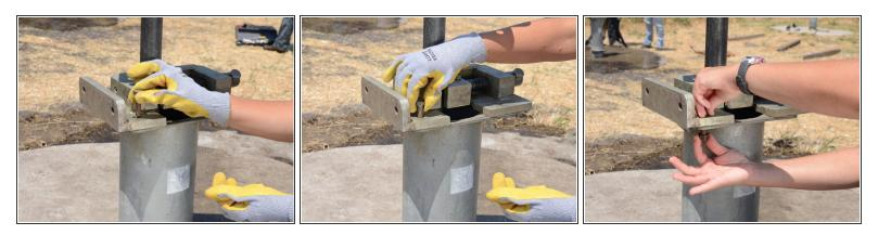
• Secure the pipe vise to the top flange with two bolts and nuts to hold the pipe vise in place.
