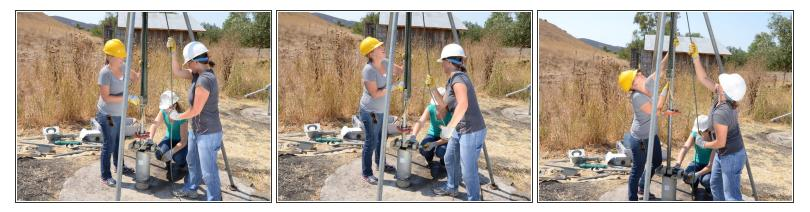
• Repeat the lifting procedure: loosen the pipe vise and pull on the rope to raise the riser main another few feet.
