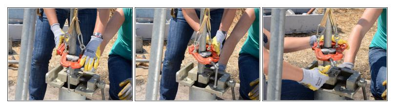
• Secure the tripod pipe vise to the riser main pipe and tighten it securely.
