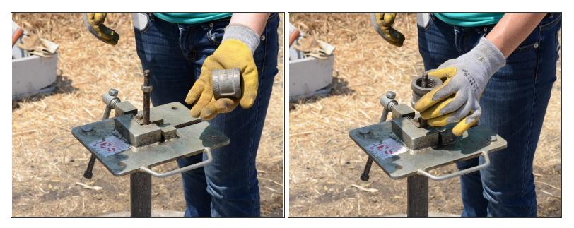
• Place a coupling over the pump rod, on top of the rod vise.
