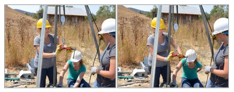
• Lower the tripod pipe vise down to the bottom of the exposed section of riser main pipe.
