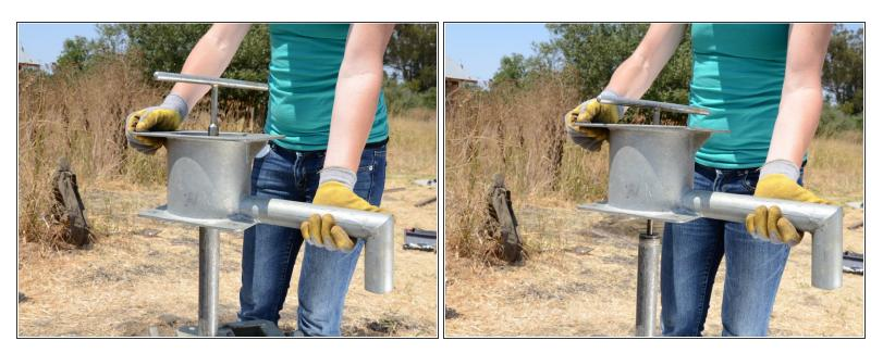
• Lift the tank up a few inches above the top of the riser main.
