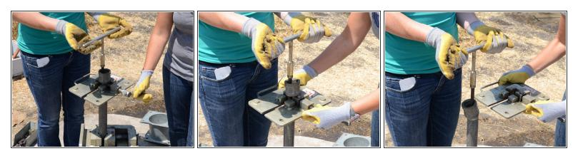
• Loosen and remove the rod vise from the pump rod.
