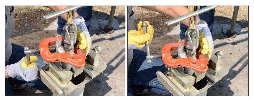
• Tighten the tripod pipe vise.
