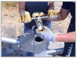
• While one person lifts up on the T-handle, remove the bolt and connection pieces.
