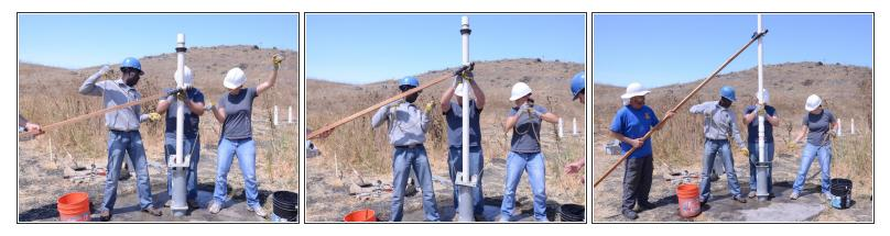
• Continue lifting the casing, supporting the top portion with the casing support, as needed.
