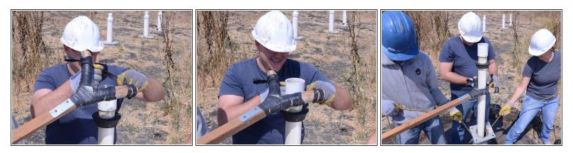
• Slip a casing support over the casing.
