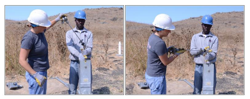
• While holding the pump rod below the first connection tightly, lower the first portion of the rod to a horizontal position.
