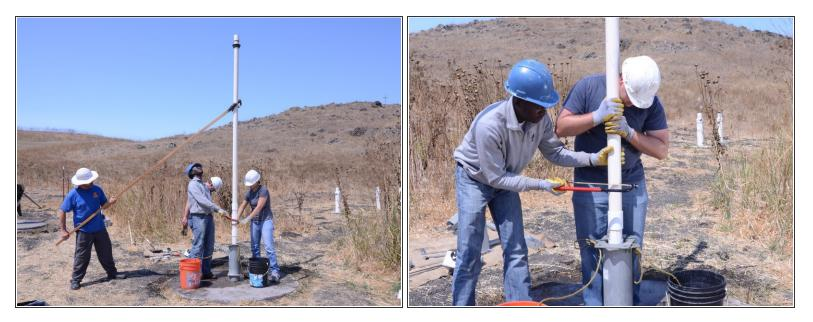
• While supporting the casing, make the necessary repairs to the casing pipe.
