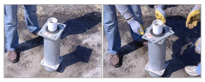
Slightly twist the head flange until the corners overhang the top of the tank, far enough so that you can grab them.
