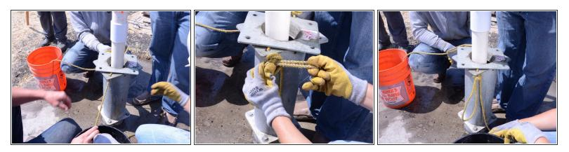
When you reach the portion of the casing that needs to be repaired, tie the casing support ropes onto the frame.
