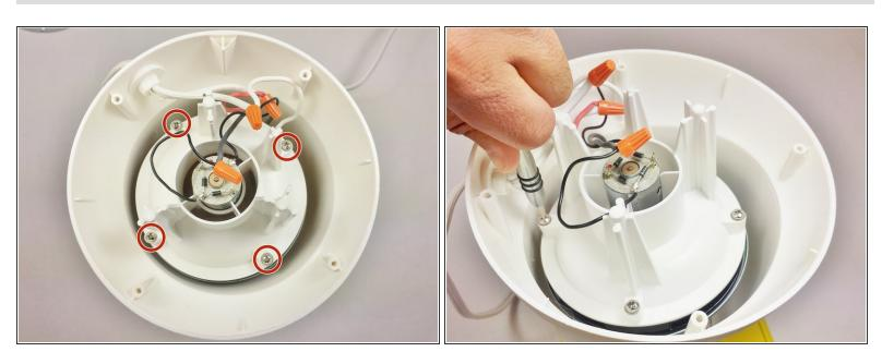
Unscrew the four 13mm Phillips #2 screws but do not remove completely just yet.
