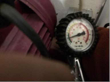
• With a compressor or even foot pump produce about 1.5 bar pressure in the boiler. There should be no water in it. Then re-open the supply and take the House water system in operation. Possible must be drawn on a \$!^&\* to fill the pump a little water.
