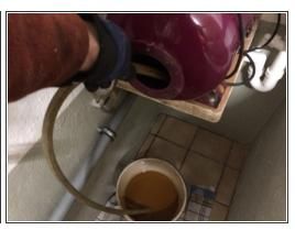
Remove the water bag. Now is still the remaining water from the leaky water bag in the boiler. With a hose through the rest of the water suction vacuum.
