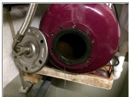
Loosen the screws with a 13 mm ring spanner, caution it runs out the water. Best to make a bucket to catch the water including. Then remove the cover. You can see the old bag. This can now be removed. The water bag is very dirty, therefore it is recommended to dress gloves
