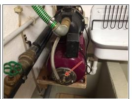
• Install the new water bag and then screw the lid. The screws should be not to tight. Please make sure that the water bag is properly seated. Usually this is more curved on a page, this page comes down.
